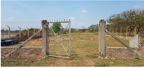
Figure 4. Wastewater Treatment Plant (WWTP) in Montero, with area for burial of dry solids. Storing of covered containers in prior to burial (to the left). Source: (Y. Geber 2019).
