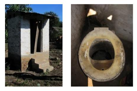
Figure 36. Toilets in Saveedra lacking in maintenance. Left photo shows toilet with broken door and right photo shows a dirty, broken toilet ring.
