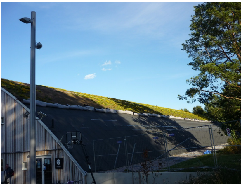
Figure 2: A green roof is being rolled onto a curve-shaped building in Uppsala, Sweden. (Photo: P. Sjöholm 2013)
