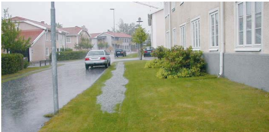
Figure 1. Locally handled storm water during a heavy rain (Göran Lundgren 2007).
