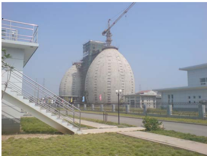
Figure 17. Biogas facilities under construction at San Jin Tan WWTP.
