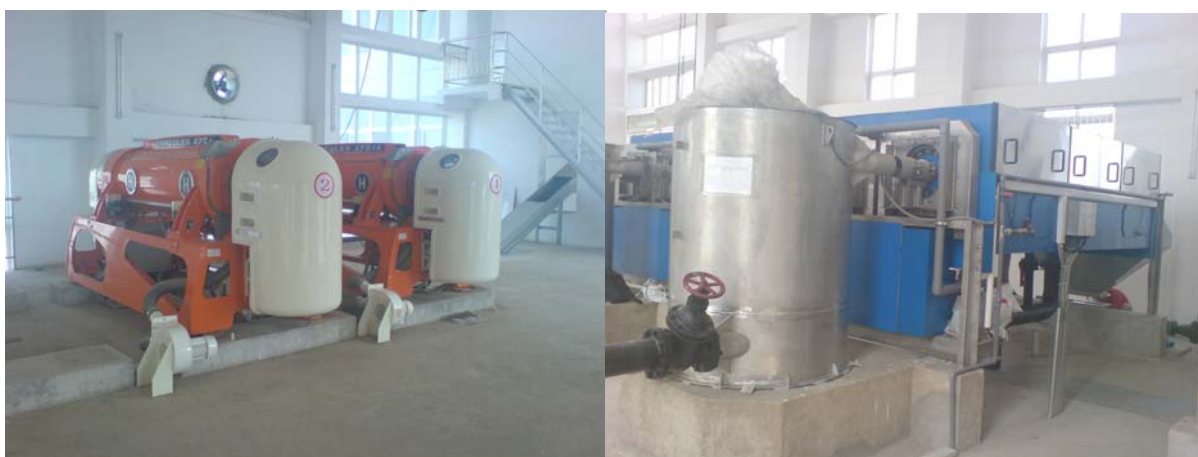
Figure 16. Dewatering centrifuges (left), drum thickener (right) at San Jin Tan WWTP.
