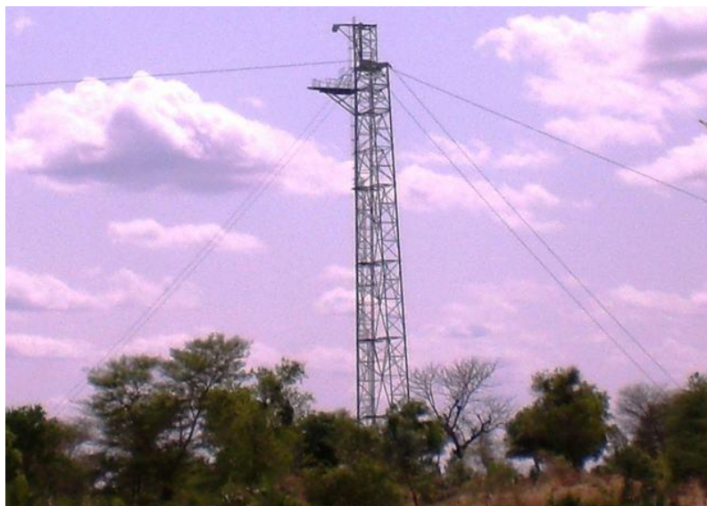
Figure 2 Right bank tower of the cable way at El Deim station. (Wilson, 2008)
