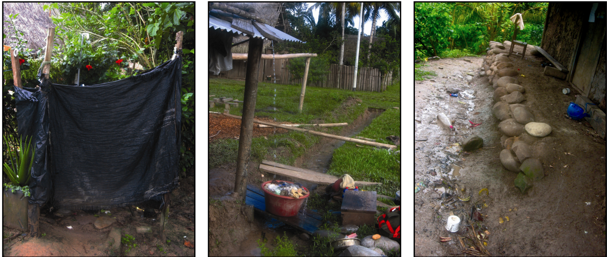
Figure 14 Standpipe used as shower (left) and for laundering (middle); unhygienic conditions resulting from the lack of stormwater management (right).
