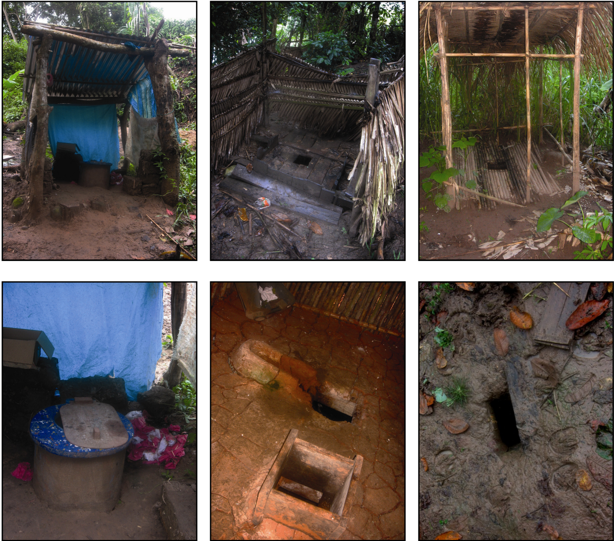
Figure 13 Common latrine superstructures and different types of user interfaces.
