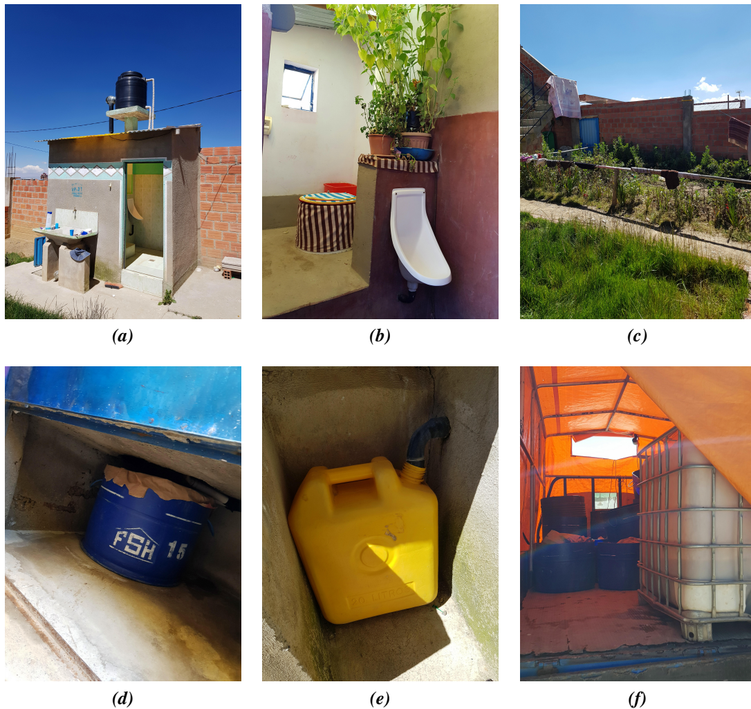
Figure 8: User interface, collection and storage/treatment phase and conveyance phase of the UDDT system. (a) The most modern bathroom with a UDDT constructed under governance of the FSH is named MOSAFA-ECO. (b) Urine and faeces are separated in a UDDT or in a urinal. (c) Ornamental plants in a greywater garden. (d) Mobile recipient for faeces collection and storage. (e) Jerrycan for collection and storage of urine. (f) A vehicles that in conveyance phase transport urine in a tank and faeces in mobile recipients.
