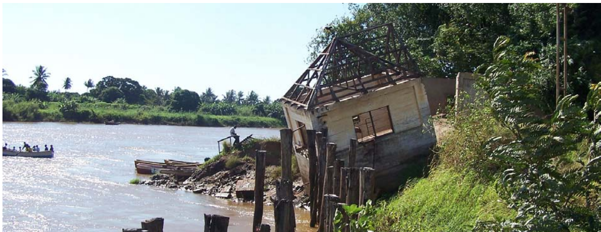
Figure 6.12. Erosion can cause a collapse of the river bank and this house was destroyed by the last flood. The poles are placed to prevent more erosion and houses from getting caught by the river (Photo Lovisa Lagerblad).
