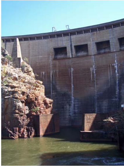
Figure 4.4. Chicamba Dam from below. Two turbines can produce a maximum of 19.2MW each (Photo Lovisa Lagerblad).
