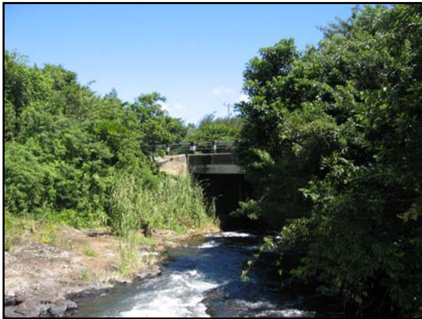
Figure 5 The bridge at River Cascades, sampling site Redit.
