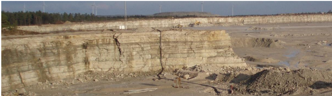
Figure 1 Picture overlooking a part of the Klinthagen quarry, notice the stratified rock composure. The rock wall is about 15 meters in height.
