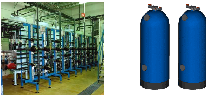
Figure 2: Mercatus' ion exchange (Mercatus, 2007) equipment to the left and Vilokan's EnvoChange ion changer to the right (Vilokan, 2007).
