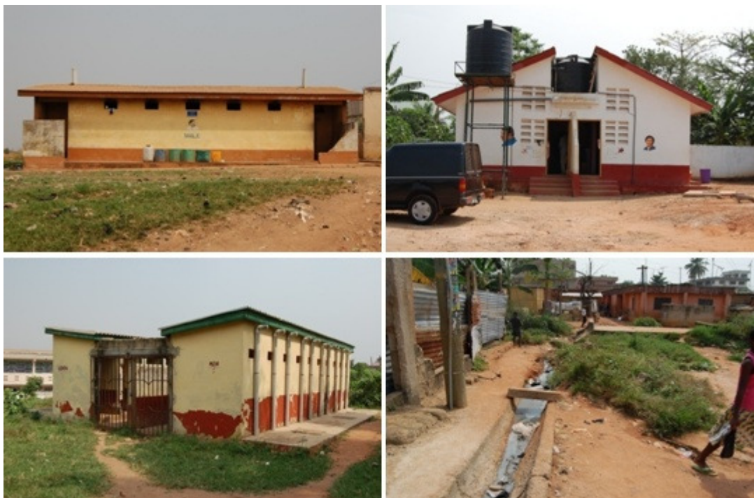
Figure 5 Public toilets vary in standard and price. Top left: public pit latrine. Top right: public WC, with a fee approximately 10 times higher than for the pit latrine. Bottom left: school KVIP. Bottom right: The open gutter system does not reach all areas. Here, the gutter ends in a residential area (author's photos).
