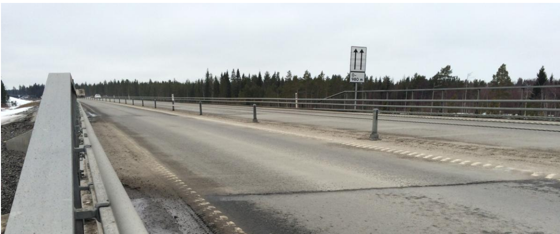
Figure 8. Road E12, contract 5 in the Umeå project. Photo: Katarina Wärmark.
