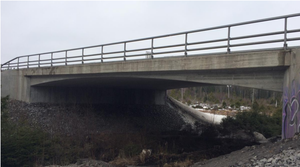
Figure 7. Bridge at the road E12, contract 5 in the Umeå project. Photo: Katarina Wärmark.
