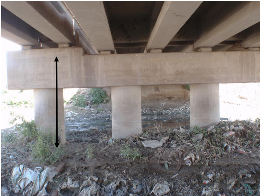
Figure 25 Historical water level mark on the Cotapachi Bridge, measured to 3 meters.
