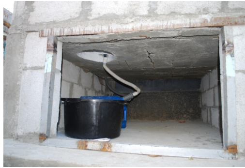
Figure 11 Compartment underneath the toilet. Urine is collected in the tank connected to the hose and faeces in the black container (photo by Katja Larnholt).
