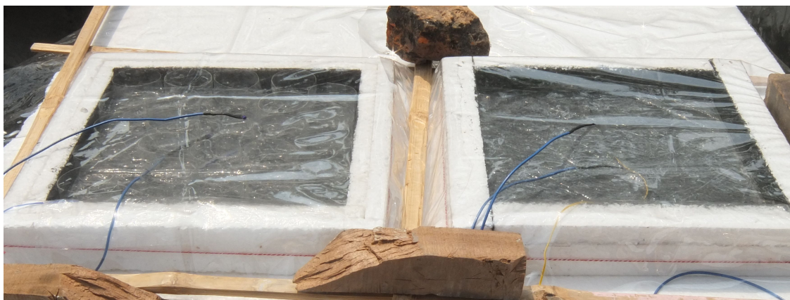
Figure 10 The performance of solar heating test with double insulation and single air gap compared with double air gap. Here the two test devices are set with thermometers and polyethene sheets on top ready for measurement.
