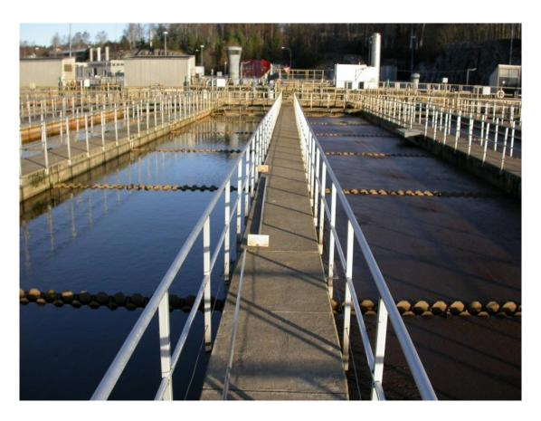
*Figure 12.* The experimental and control line. The surface of the control line (right) is covered with sludge, and the experimental line (left) has a clear surface of water.
