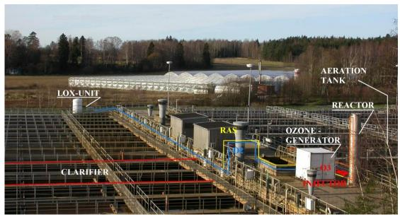
Figure 11. The experimental plant at Himmerfjärden WWTP.
