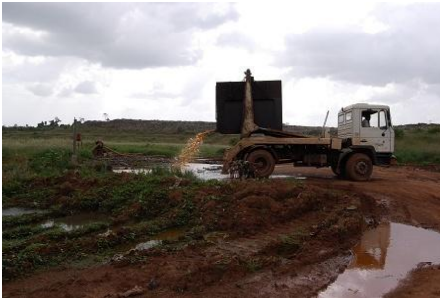
Figure 13 Emptying of fecal sludge in the first pond for co-treatment of landfill leachate and fecal sludge. The landfill is seen in the background.
