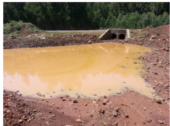
Figure 17. The water of site N was linked with a ditch on the other side of the road through a concrete culvert (Carlström, 2013)
