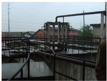
Figure 27: One of the two SBR tanks.
